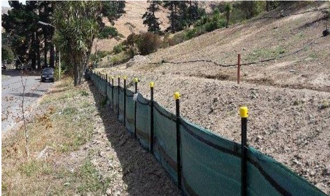
Figure 3: Typical example of sediment fence
