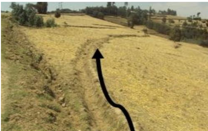
Figure 4: Typical cut off drain on site
