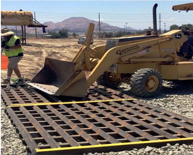
Figure 1: Typical example of stabilised construction exit
