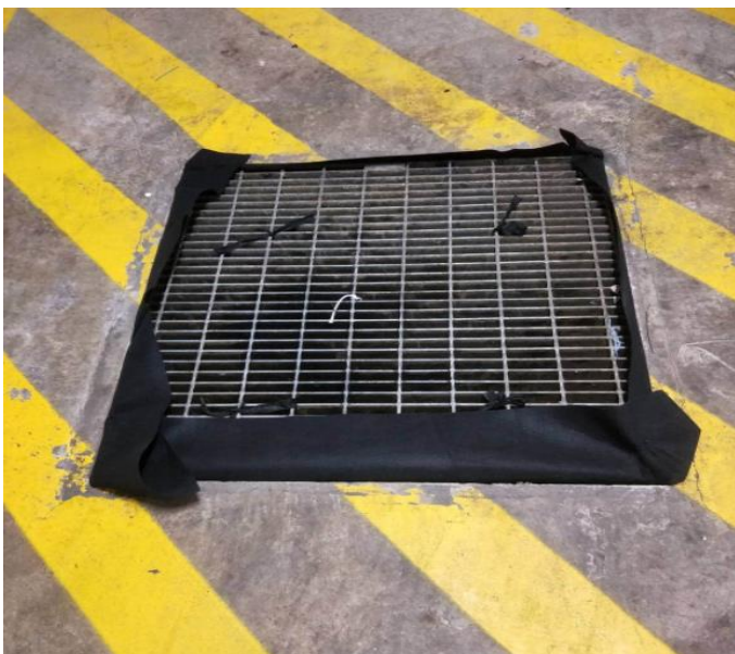
Figure 10: A typical surface inlet trap
