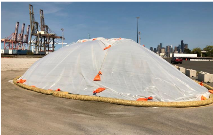
Figure 6: Stockpile covered on site
