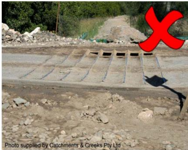
Figure 2: Lack of maintenance resulting in heavy sedimentation
