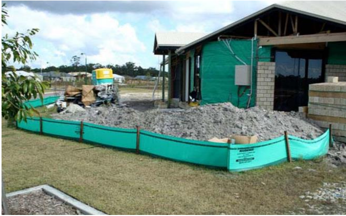
Figure 5: Stockpile surrounded with a sediment fence
