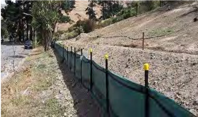
Figure 3: Typical example of sediment fence
