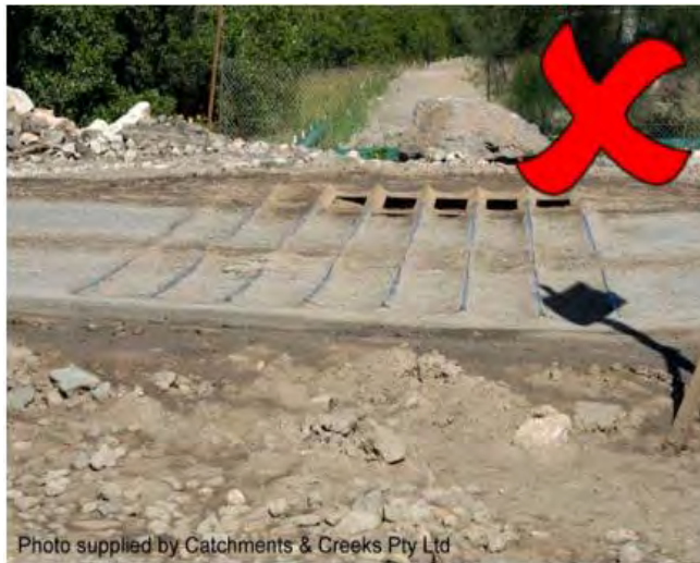
Figure 2: Lack of maintenance resulting in heavy sedimentation
