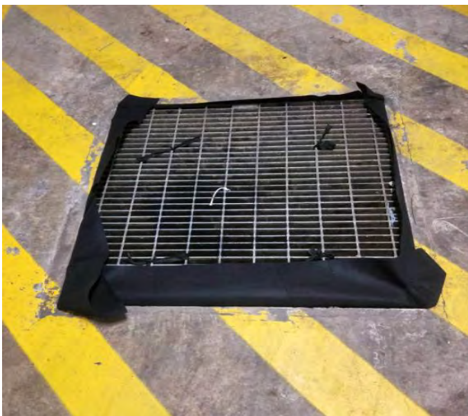
Figure 10: A typical surface inlet trap
