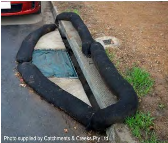
Figure 9: Use of filter socks to form a sediment trap at sag inlet
