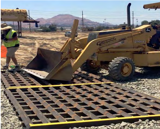
Figure 1: Typical example of stabilised construction exit
