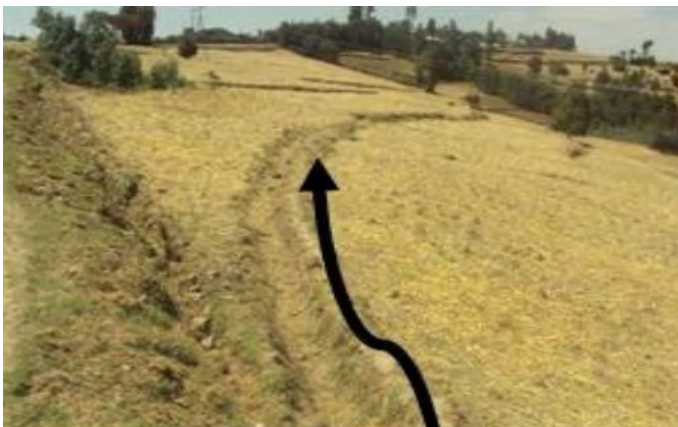
Figure 4: Typical cut off drain on site
