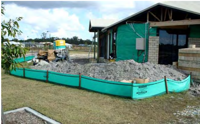
Figure 5: Stockpile surrounded with a sediment fence
