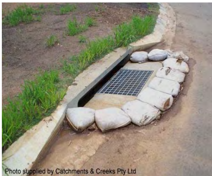
Figure 7: Typical example of sandbags surrounding a kerb inlet pit
