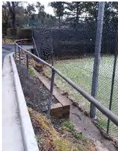
Photo 6 – Timber sleeper retaining wall
