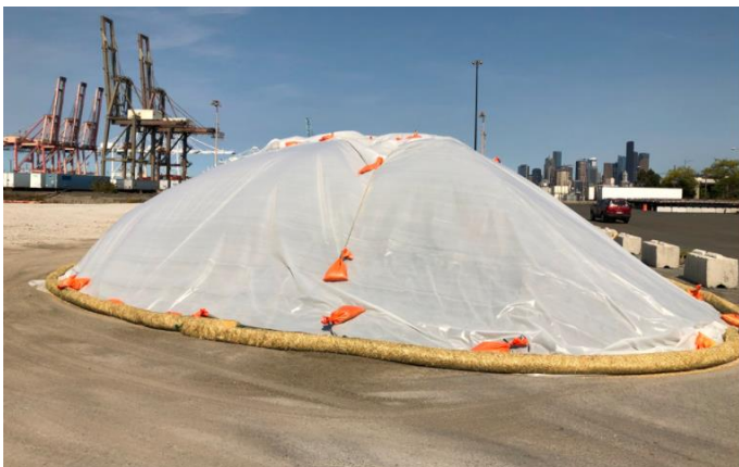
Figure 6: Stockpile covered on site
