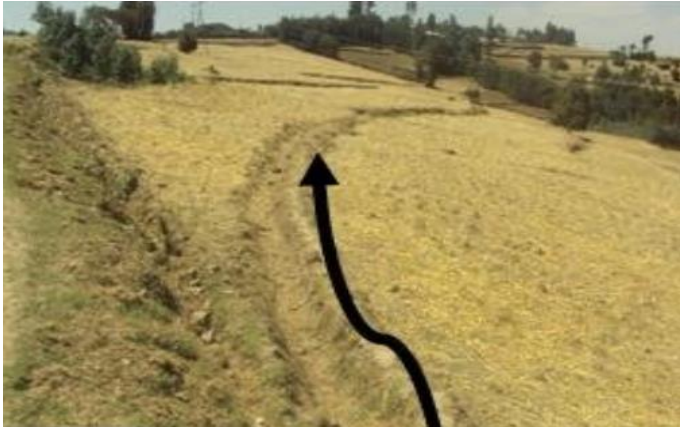
Figure 4: Typical cut off drain on site
