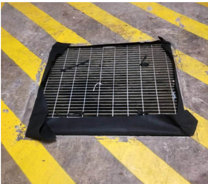
Figure 10: A typical surface inlet trap
