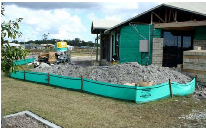
Figure 5: Stockpile surrounded with a sediment fence
