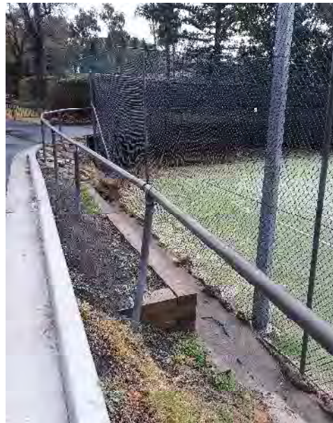
Photo 6 – Timber sleeper retaining wall
