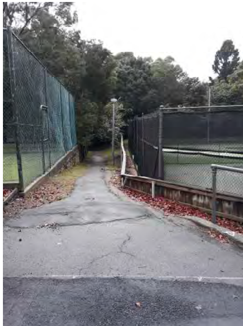
Photo 3 – Asphaltic concrete pathway
