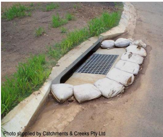
Figure 7: Typical example of sandbags surrounding a kerb inlet pit
