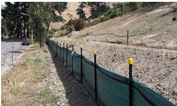
Figure 3: Typical example of sediment fence
