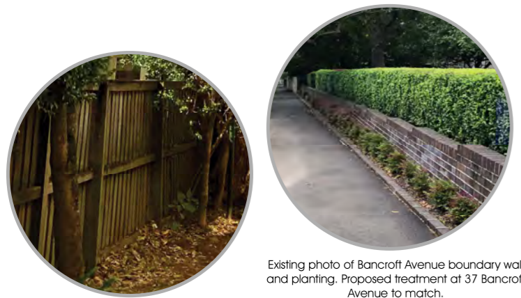
Existing photo of timber boundary fence north-south between new SWELL building and 39 Bancroft Avenue. Proposed new fence to be replaced with slightly modify detail including 3 rail, lapped and capped with metal posts.
