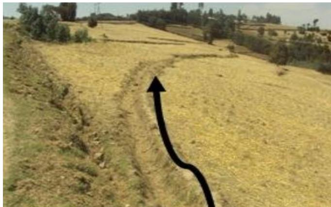
**Figure 4: Typical cut off drain on site**
