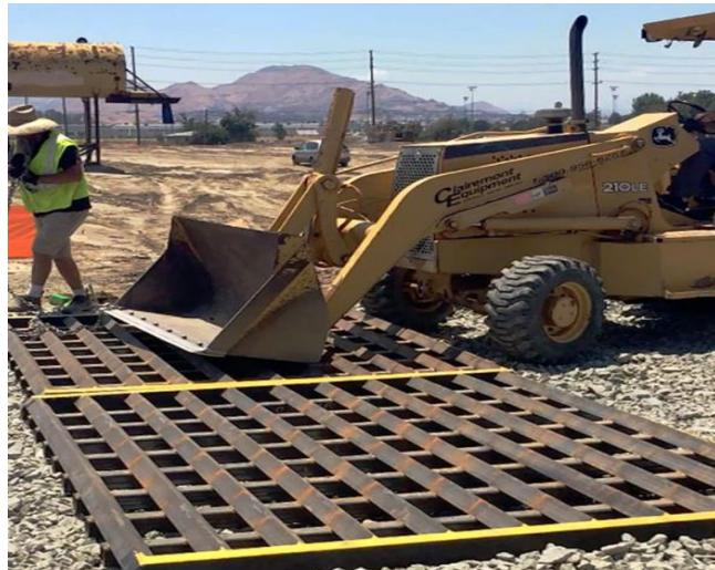
**Figure 1: Typical example of stabilised construction exit**
