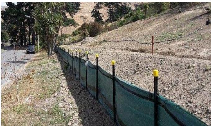
**Figure 3: Typical example of sediment fence**
