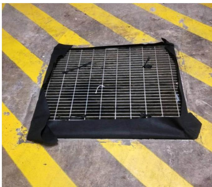
**Figure 10: A typical surface inlet trap**
