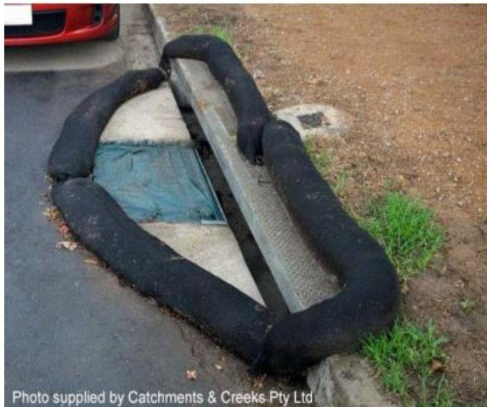
**Figure 9: Use of filter socks to form a sediment trap at sag inlet**
