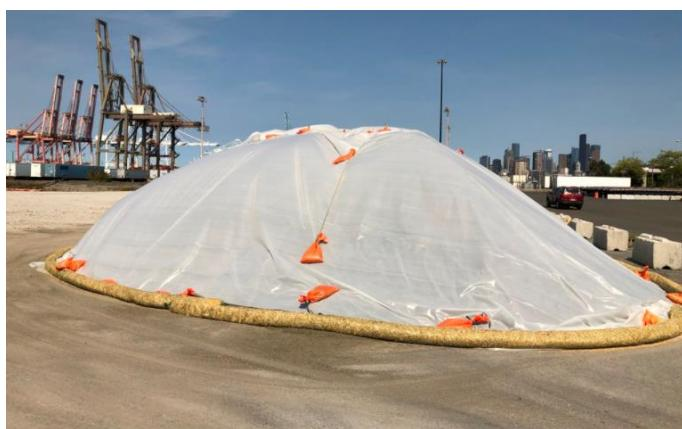
**Figure 6: Stockpile covered on site**
