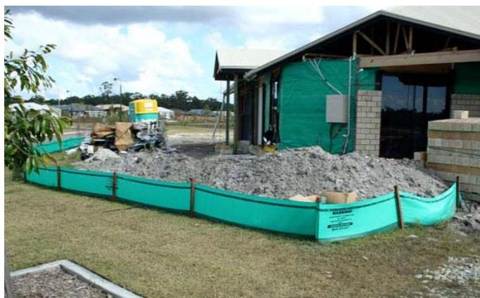
**Figure 5: Stockpile surrounded with a sediment fence**
