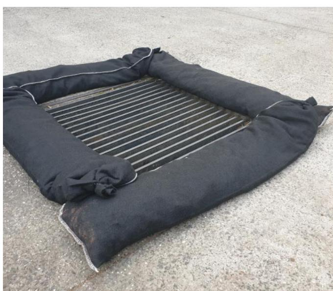
**Figure 8: Sandbag sediment trap other than kerb inlet pit**
