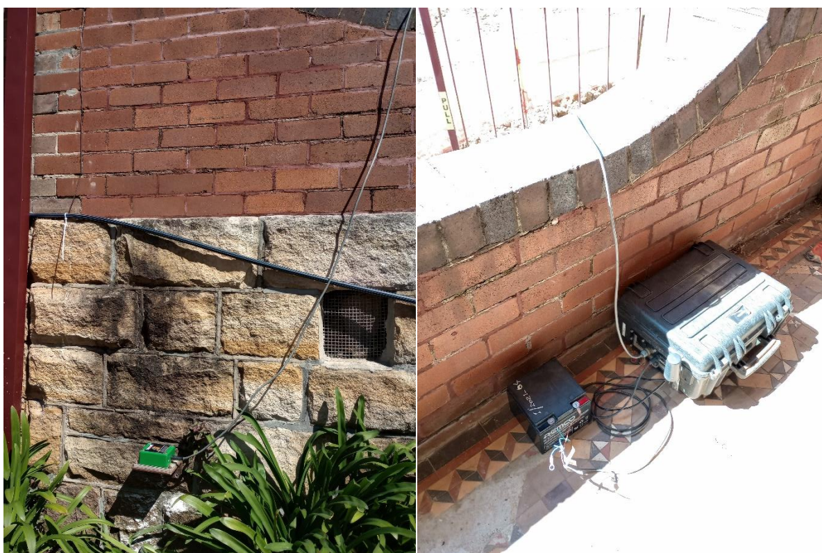
Figure 2: M7427 at the front area of the heritage building
